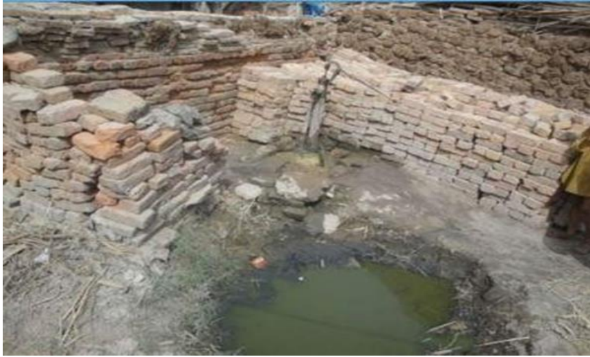
Fig 4: showing Poor drainage causing groundwater contamination.
